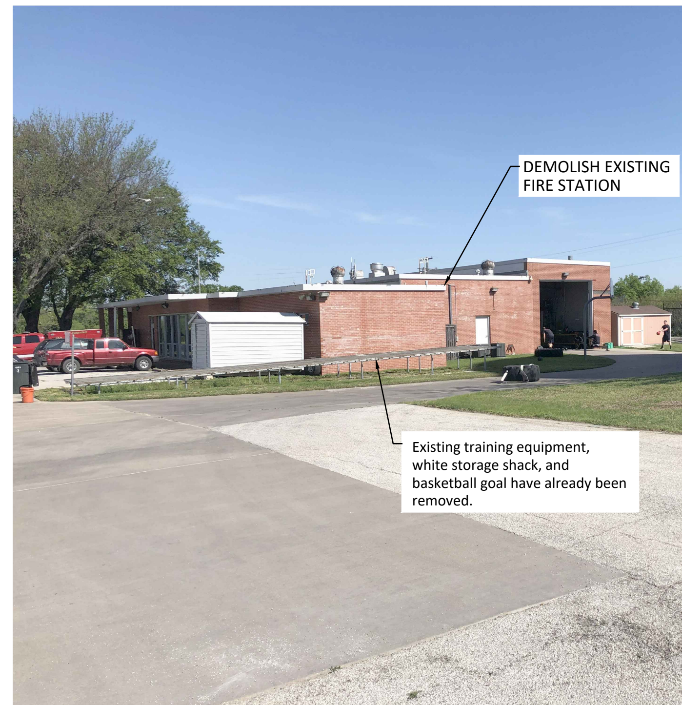
2 FIRE STATION #3 (BACK VIEW)
