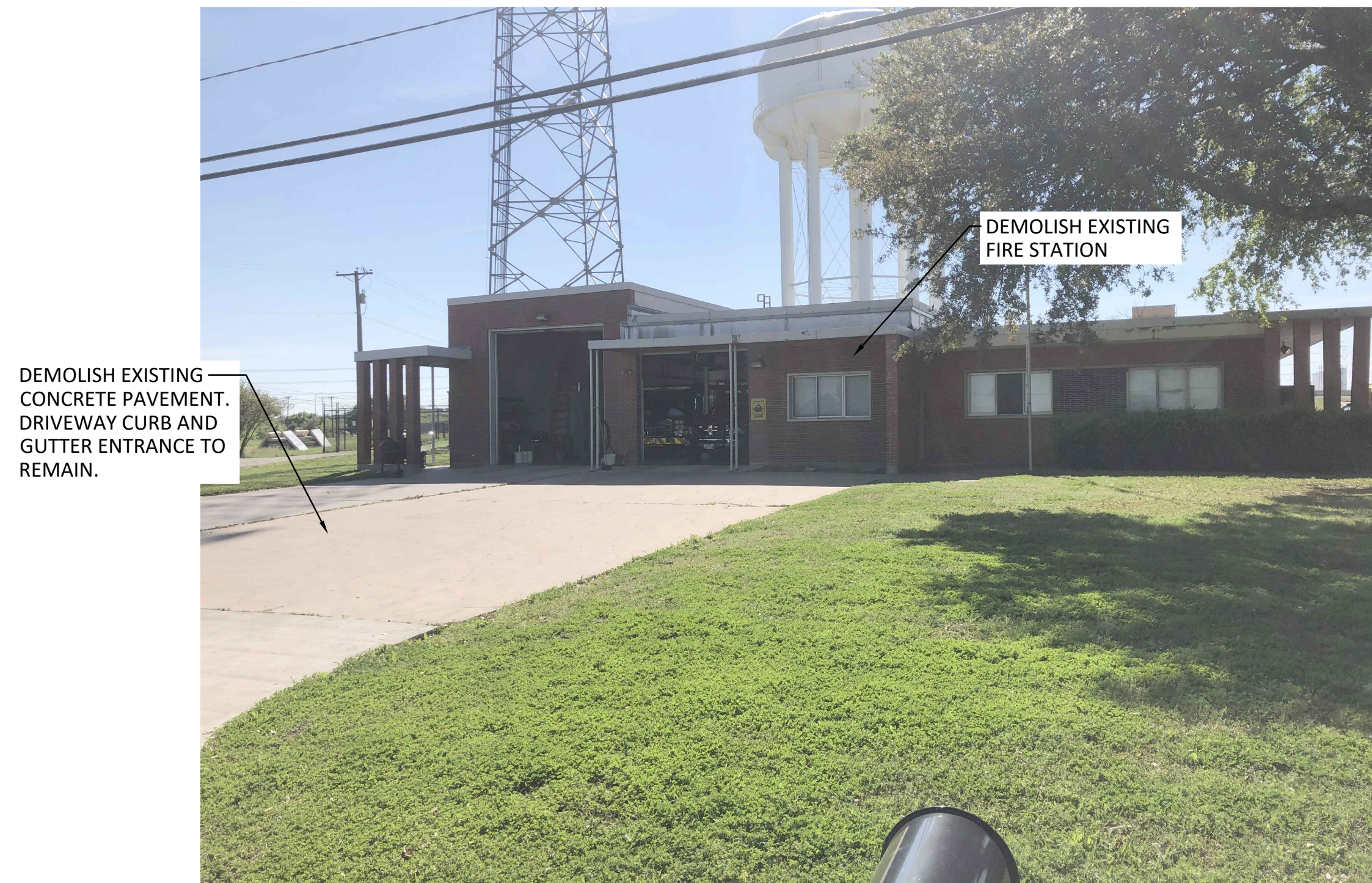
1 FIRE STATION #3 (FRONT VIEW)
